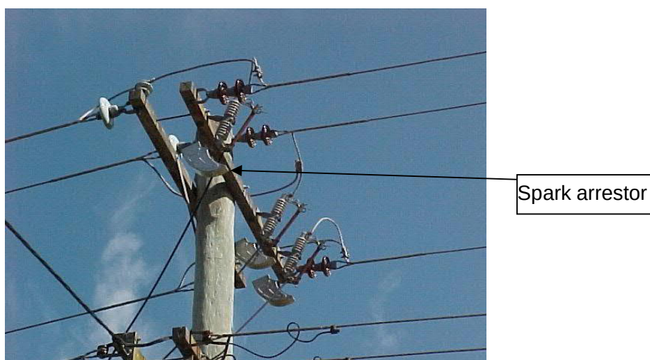
Figure 14: Dropout fuse spark arrestor
