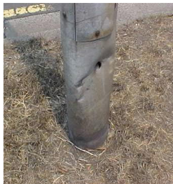
Figure 8: Vehicle Impact damage
