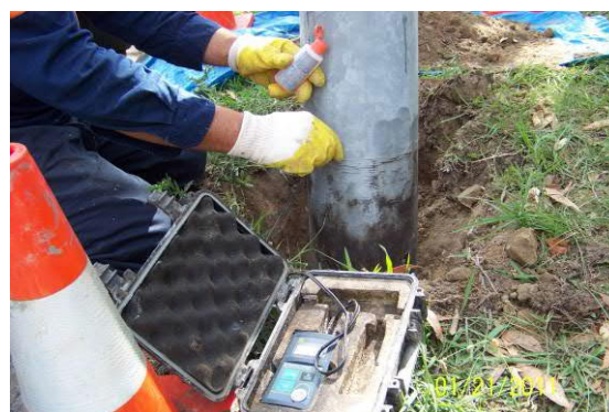
Figure 26: Testing the wall thickness
