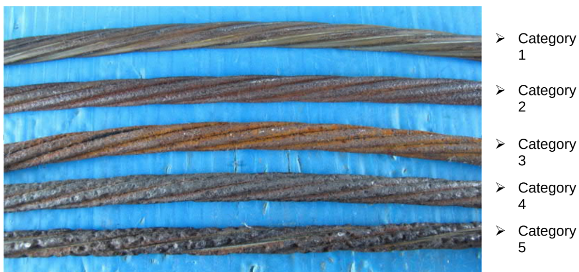
Figure 16: Steel conductor condition/corrosion categories
