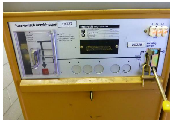
Figure 6 – CI1 operating mechanism
