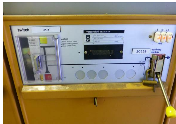
Figure 5 – CIT operating mechanism
