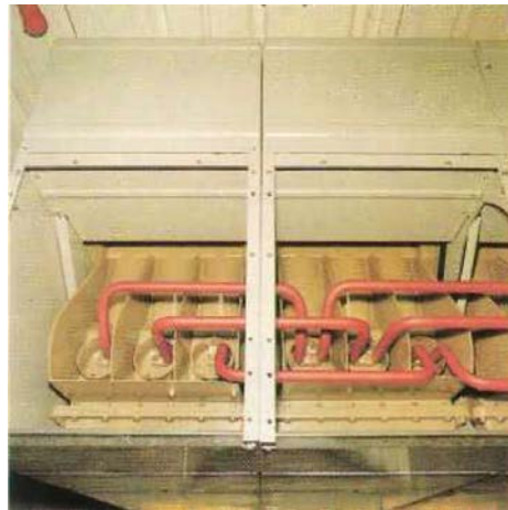
Figure 4 – Bus bar compartment
