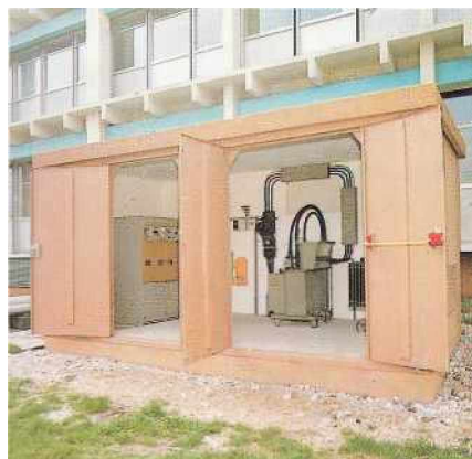
B120 transformer substation with Vercors M6 cubicles
