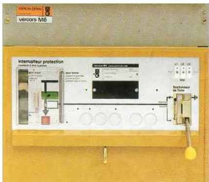
CI1 operating mechanism
