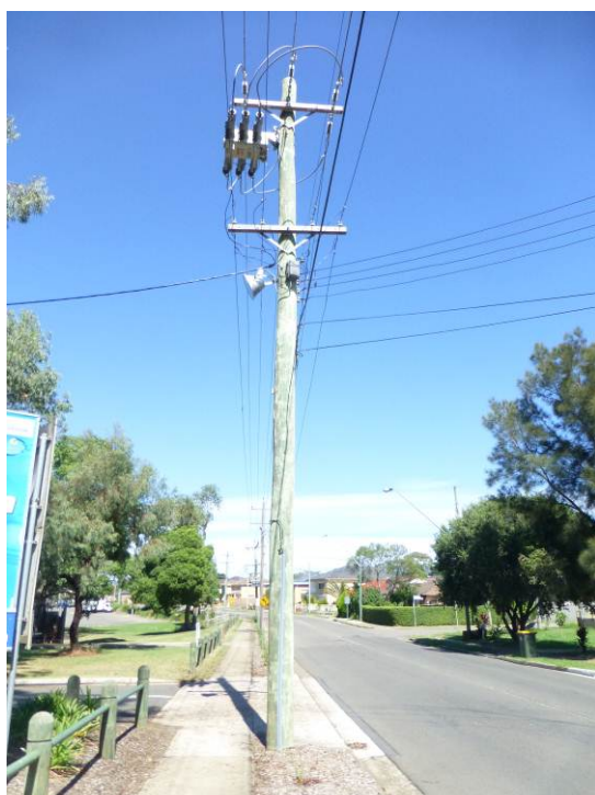
Figure 3 – Photos of an installed Iljin LBS
