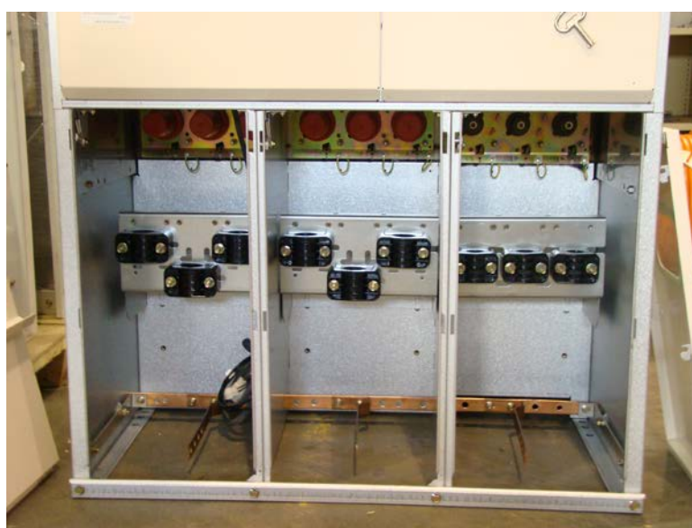
Figure 8 - Cable clamping arrangement
