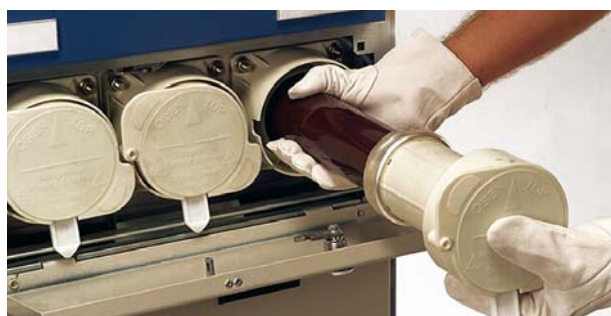
Removal of the fuse link
