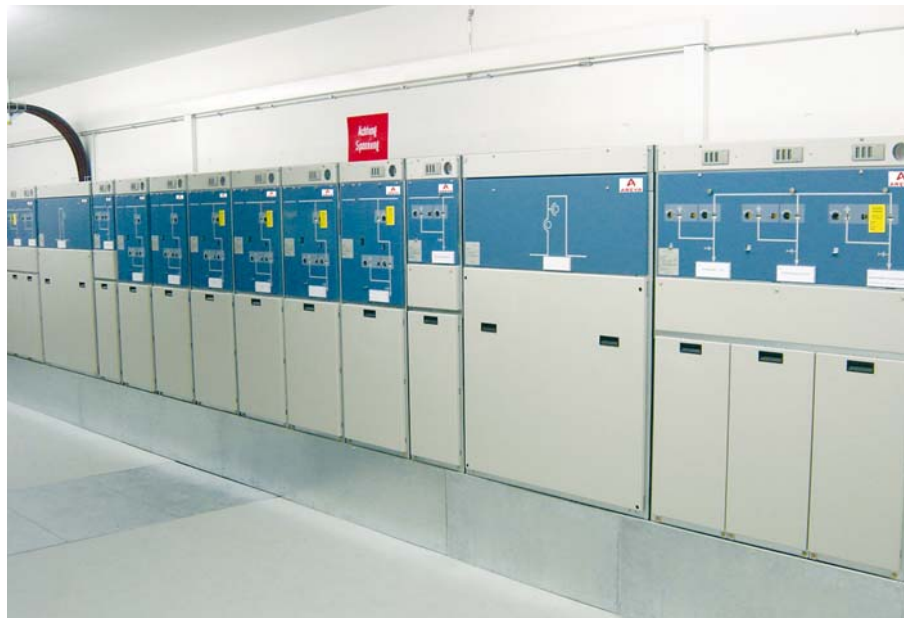
Example of an extensible FBX-E switchgear:
