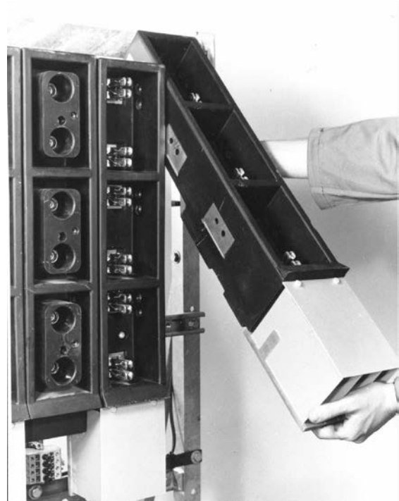
Hang fuse strip over top Unistrut support frame bracket
