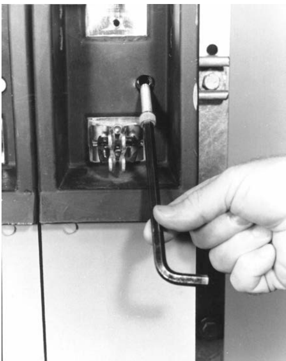
Push fuse strips together and lightly clamp bottom frame securing bolt
