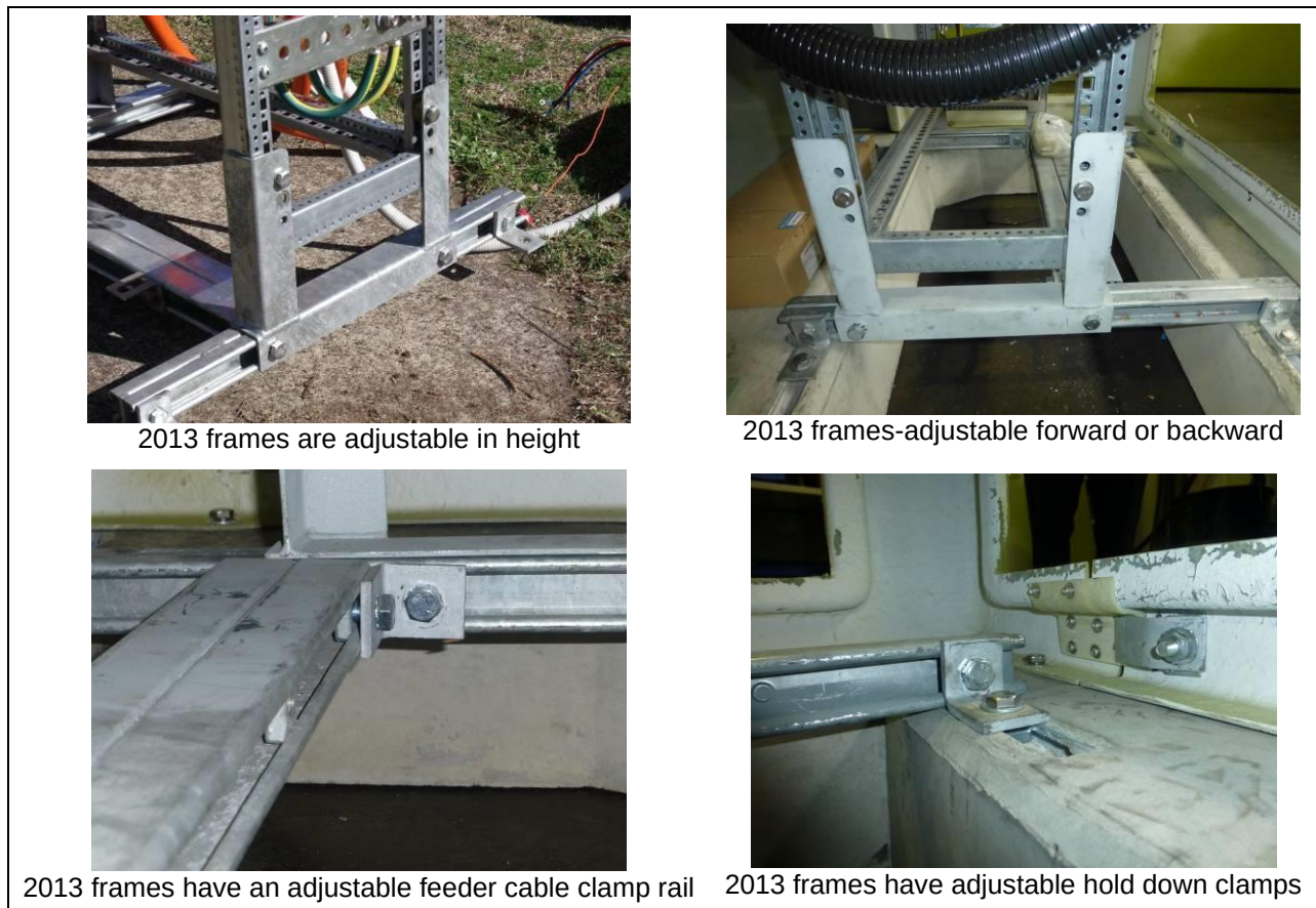
Figure 4: Adjustable mounting frames - 2013 onwards
