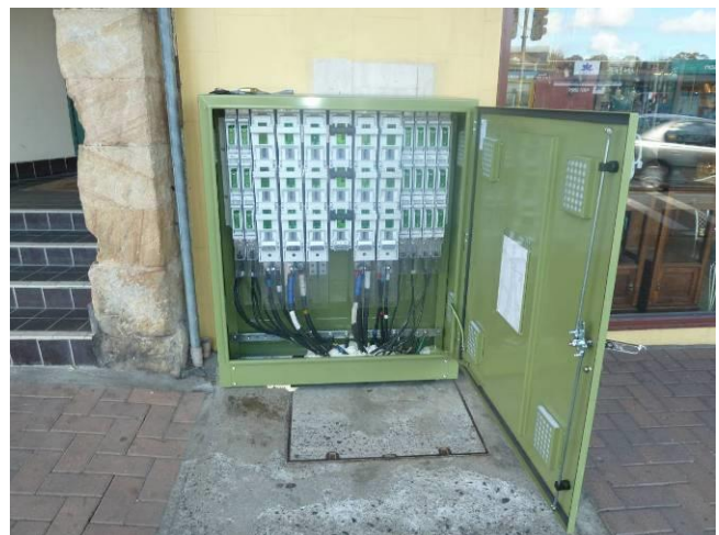
Figure 28: Example - 9 way cubicle with bus tie
