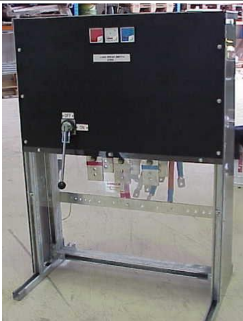
Type 3 LV LBS frame front (2100A LBS - No fuse strips)
