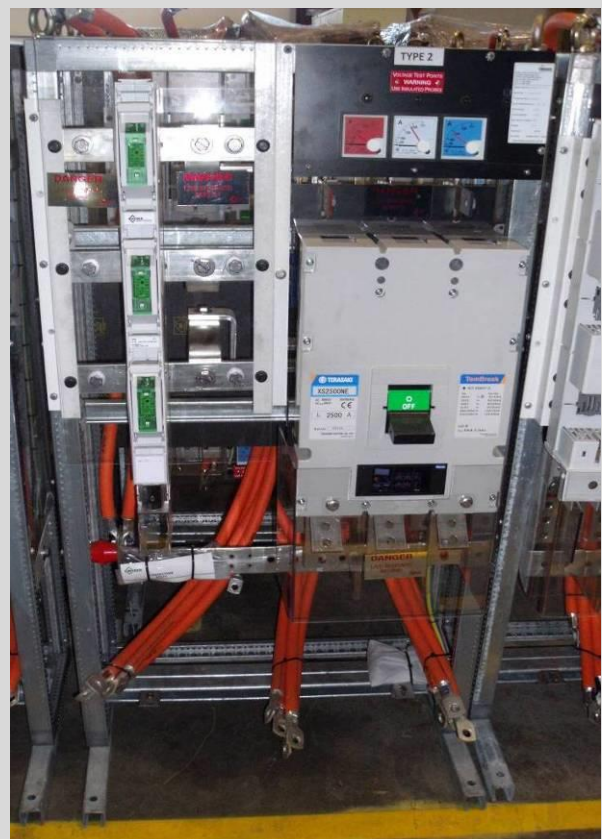
Type 2 – (Post 2013) (No switch on incomer)
