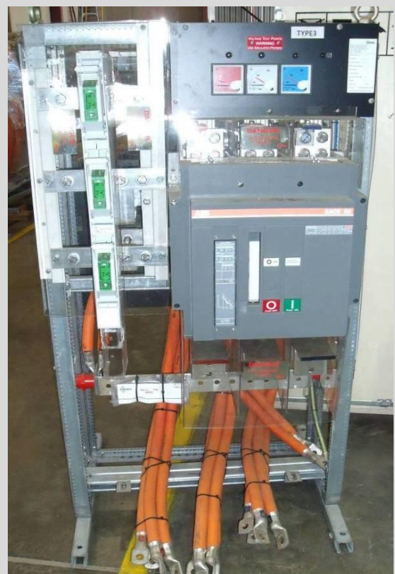
Type 3 – (Post 2013) (No switch on incomer)
