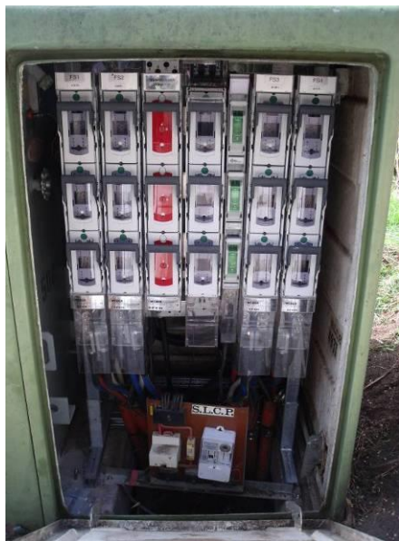
2013 Cat 1 LV board in an old narrow size 5 cubicle with switches & MDI facing the side doors
