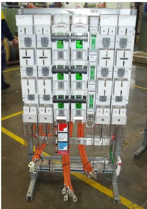
Cat 2 – (2006-2013) (With no gap between fuse strips)
