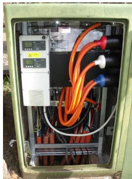
2013 Cat 1 LV board in an old narrow size 5 cubicle with switches & MDI facing the side doors
