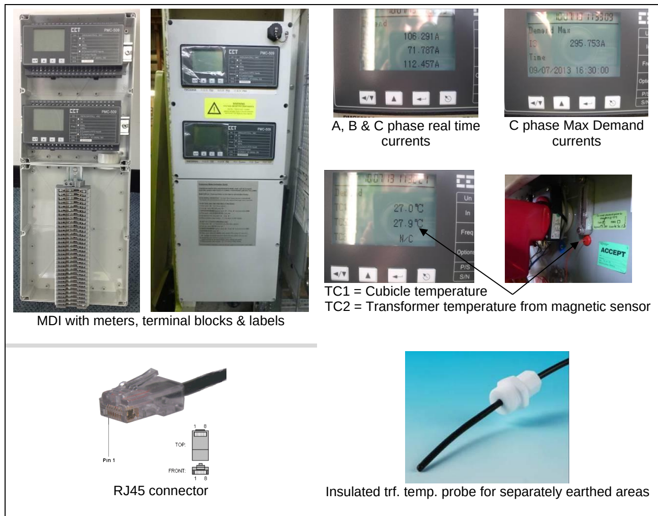
Figure 7: PMC 509 Smart MDI and components
