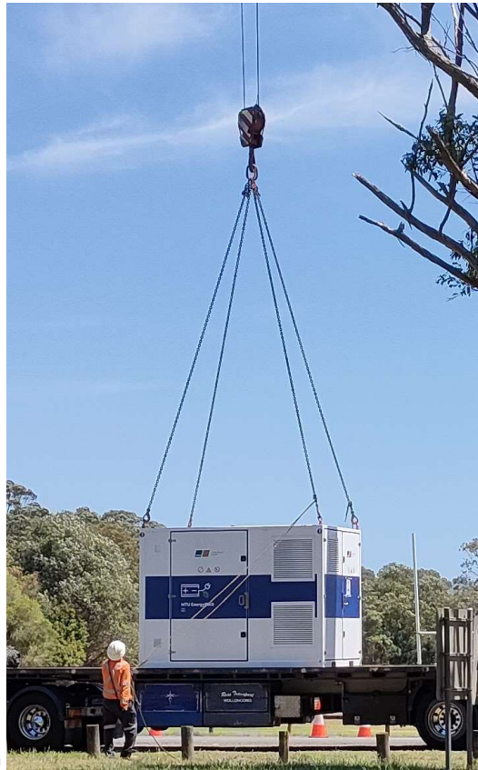
Figure 12: BESS lifting method
