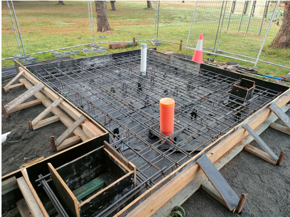
Figure 10: Foundation civil works before installation.
