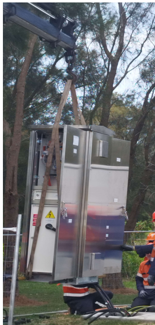
Figure 15: Lifting and installation of LV Switchboard
