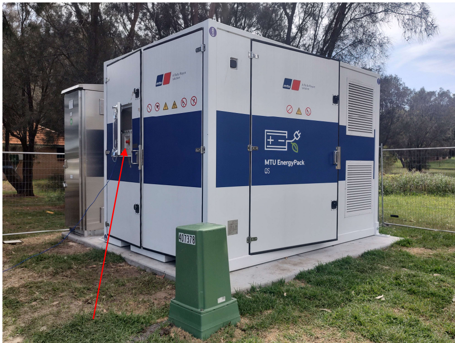
Figure 19: E-stop push button location
