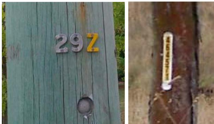
Figure 2 - Pole disc indicator and pole number plate
