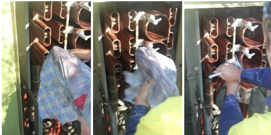
Figure 7-24: Cleaning the fixed assembly using the feather duster
