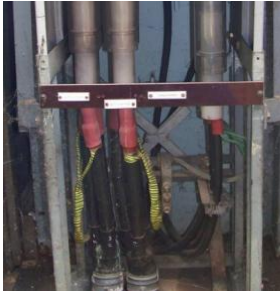
Figure 7-40: Acceptable earth connections
