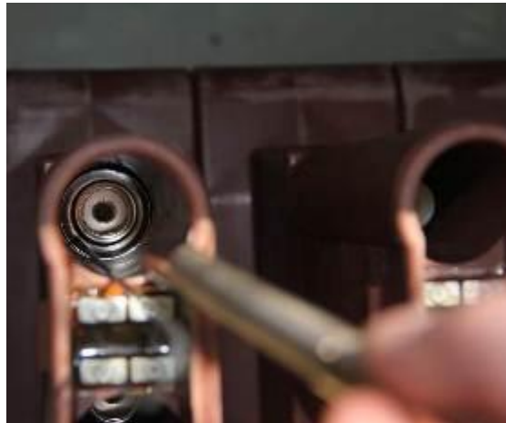
Figure 7-18: Inspection of main contact with mirror
