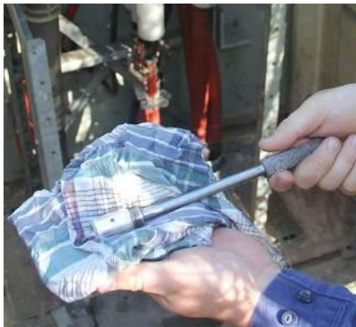
Figure 7-21: Cleaning of the main contact
