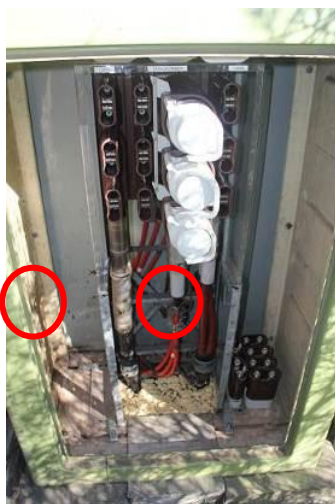
Figure 7-48: Perspex dust covered affixed using cable ties
