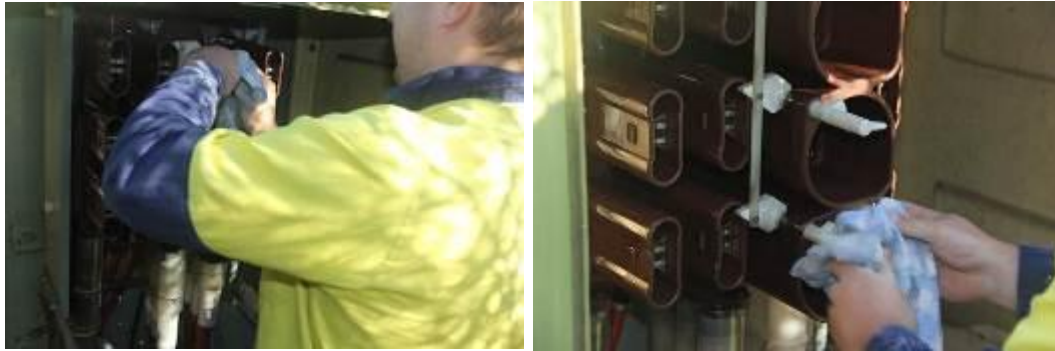
Figure 7-23: Cleaning of the fixed assembly
