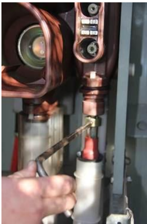
Figure 7-44: Checking the tightness of the cable connection
