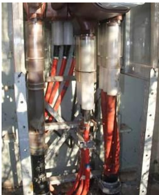
Figure 7-39: Wet termination (left) and dry termination (right)
