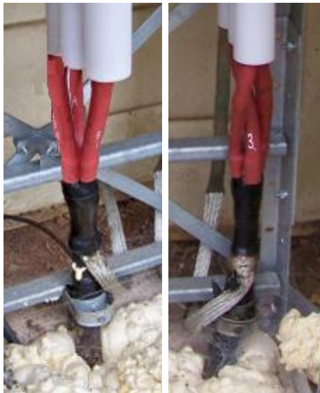
Figure 7-41: Sufficient and Insufficient cable separation
