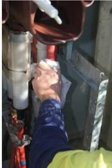
Figure 7-45: Cleaning the cables with solvent wipe
