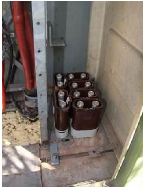
Figure 7-37: How to leave switch caps
