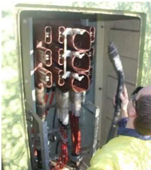
Figure 7-14: Vacuuming of HV switchgear enclosure
